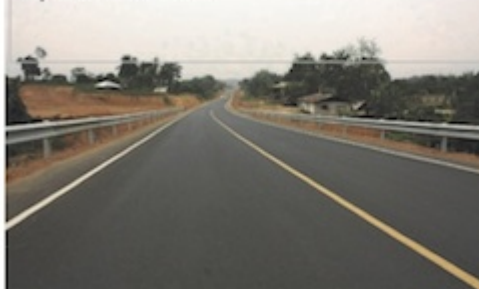
The Monrovia Redlight-Gbarnga-Guinea border Highway under construction
